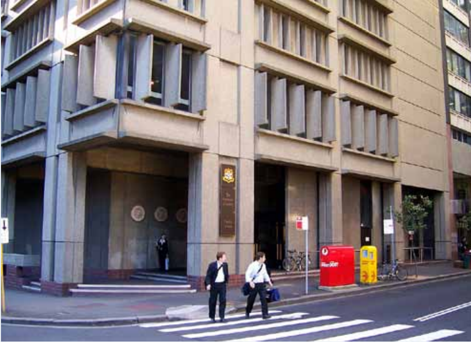
Moving in ... PIAC's new premises at 173-175 Phillip Street, Sydney.
